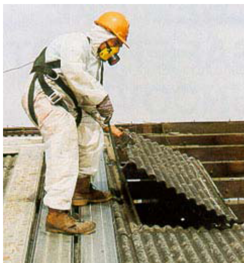
Image 106 Asbestos cement roof sheeting removal. This is an example of 'lower/minor/less significant hazard' asbestos
