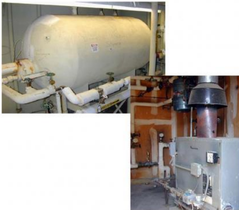
Image 105 Moulded and sprayed asbestos pipe lagging. This is an example of a potential high hazard ACM
