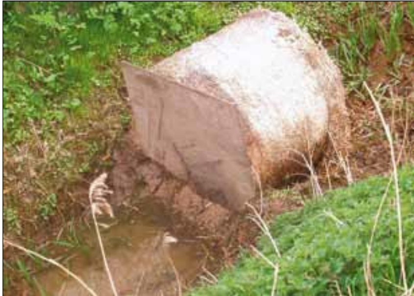
Improvised dam using soil and a hay bale.
