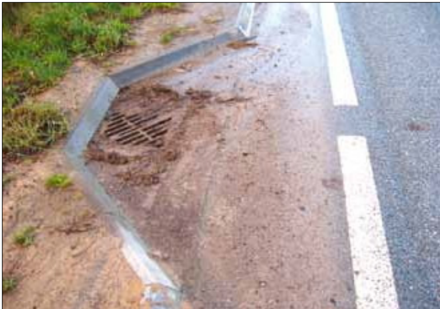
A typical road gully which can be blocked using a clay drain mat or inflatable drain blocker.
